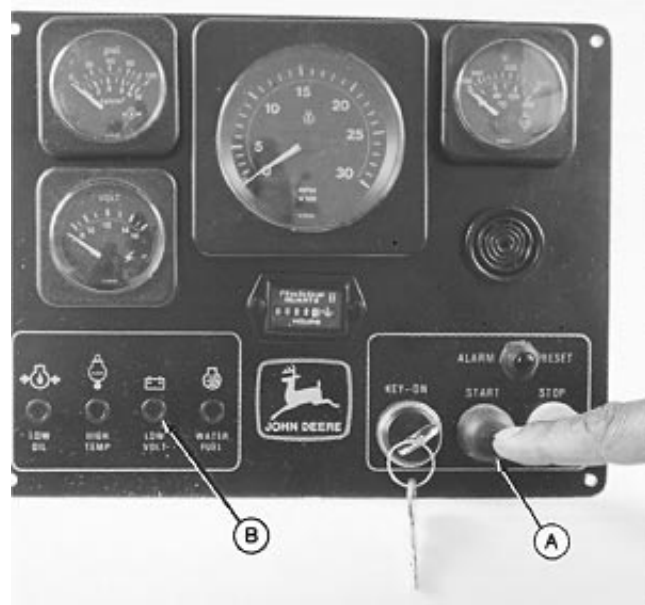
Instrument Panel - Mechanically Controlled Engines
